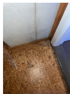
Manglende plate under sotluke.
