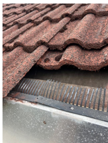
Takpapp over trebord under takpanner
